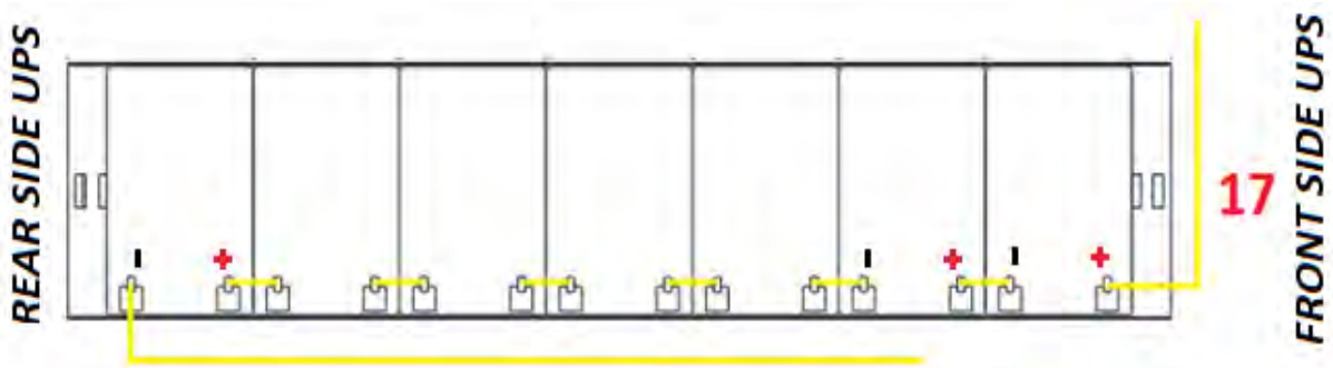
Figure 41 - View from above Level No.6 tray no. 17
