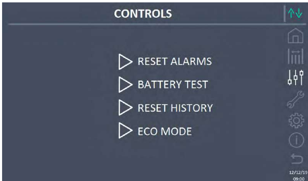
Picture 18 – Controls section
